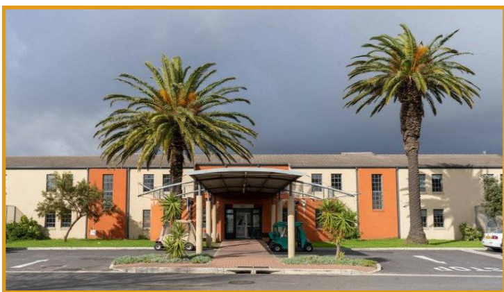
Valkenberg Hospital's new High Care Unit
